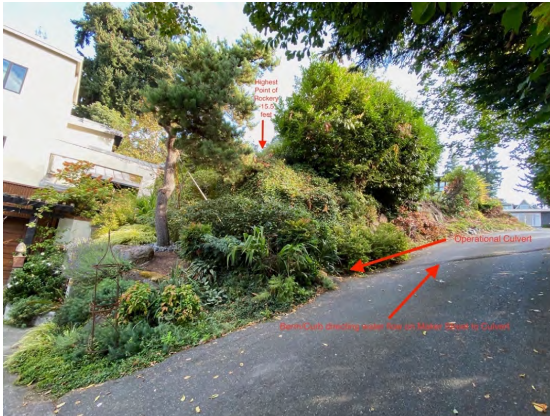
Photo of Maker Street: Looking up from house on 7030 Maker Street to adjacent uphill property, 6950 SE Maker Street. Arrows point to operational culvert and berm/curb that directs Maker Street runoff to culvert.
